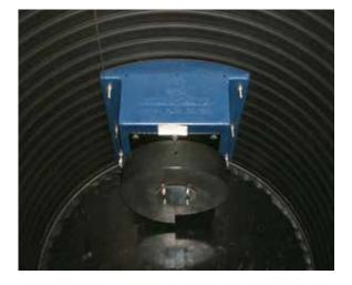
The JFC CorriFlow Chambers come complete with either a JFC Hydro-Valve or JFC Hydro-Plate which is sized to suit the design flow and design head required.
