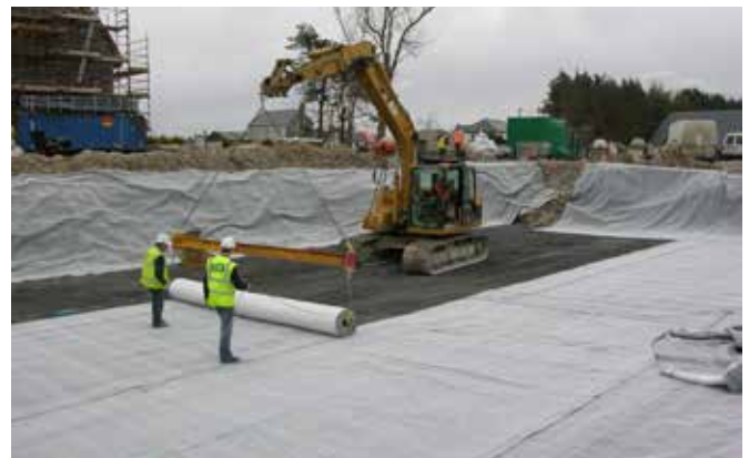
Fig. 3 – Installing GCL Liner
