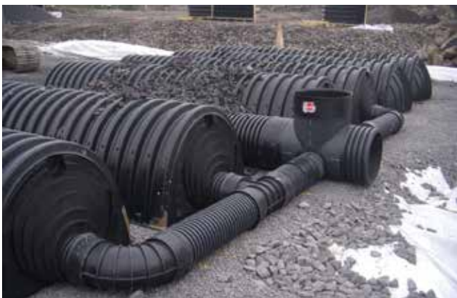
Fig. 14 –Manifold Installation
