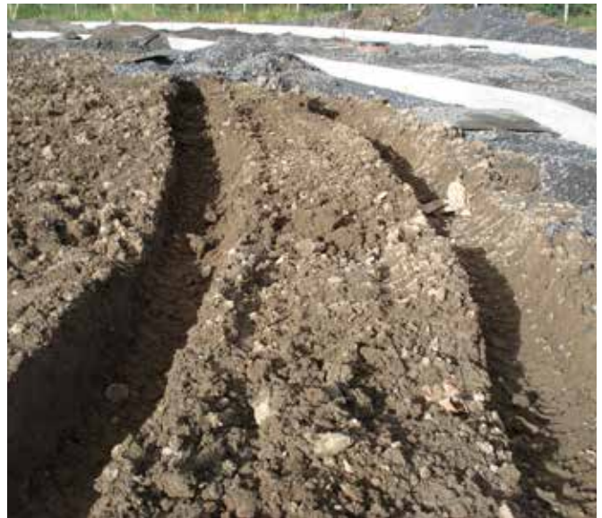
Fig. 20 – Dumper Rutting
