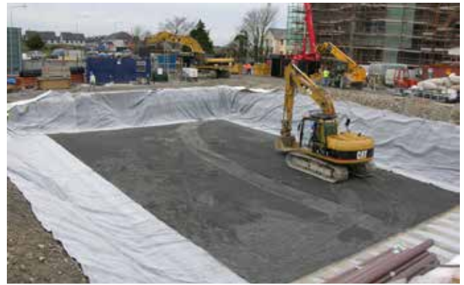
Fig. 2 – Installing GCL Liner
