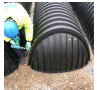
Fig. 13 – Screwing End Cap in Place
