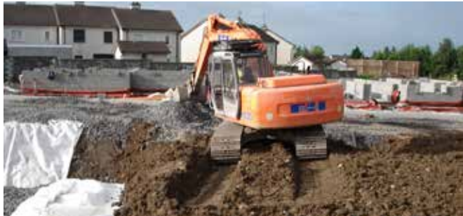
Fig. 19 – Excavator Rutting
