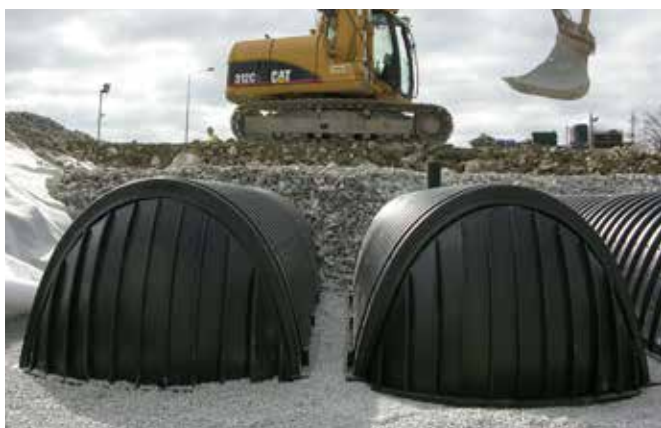
Fig. 17– Track Machine Over Chambers
