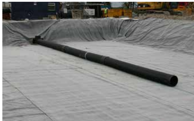
Fig. 4 – Impermeable System Distribution Pipe
