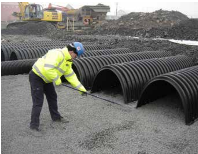
Fig. 10 – Levelling the base
