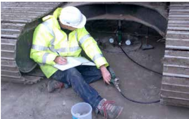
Fig. 1 – Plate Bearing Test
