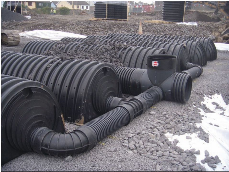
Figure 4 Typical manifold installation
