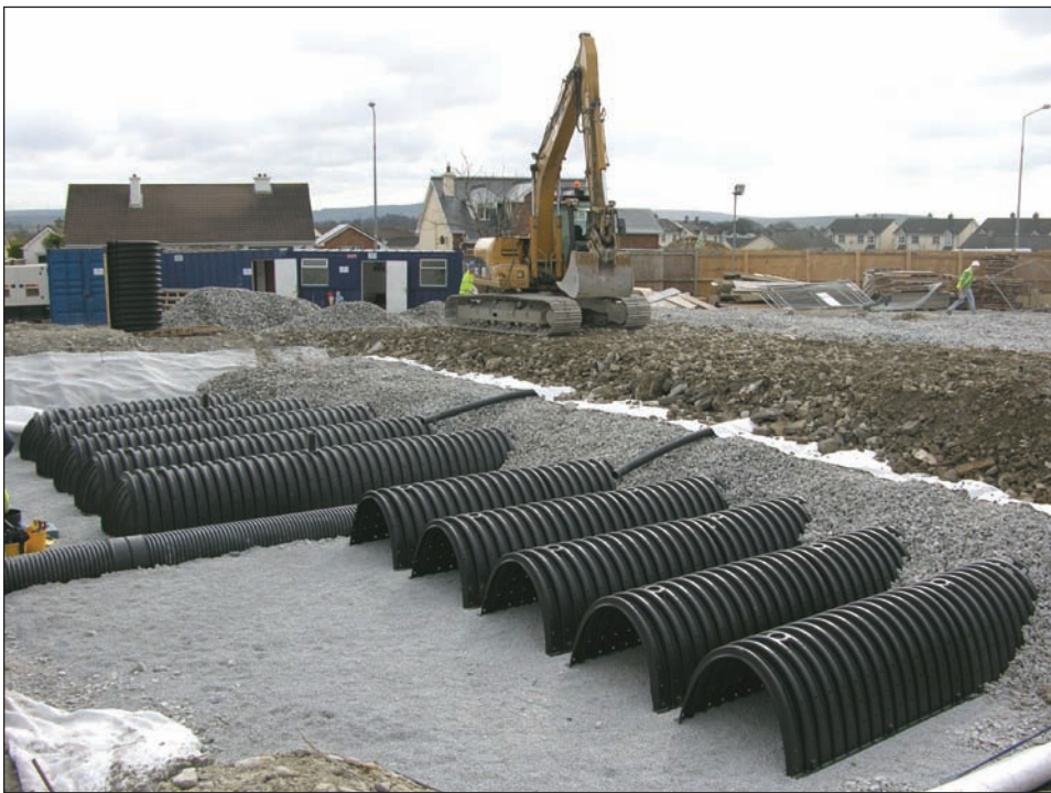
Figure 3 Typical distribution pipe installation
