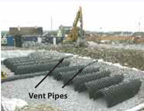
Fig. 16– Backfilling Near Completion
