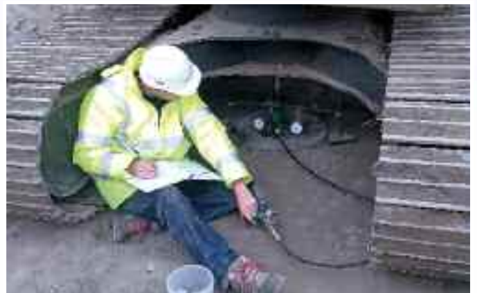
Fig. 1 – Plate Bearing Test
