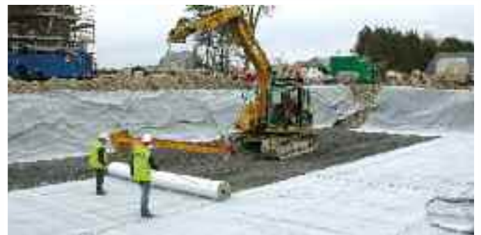
Fig. 3 – Installing GCL Liner
