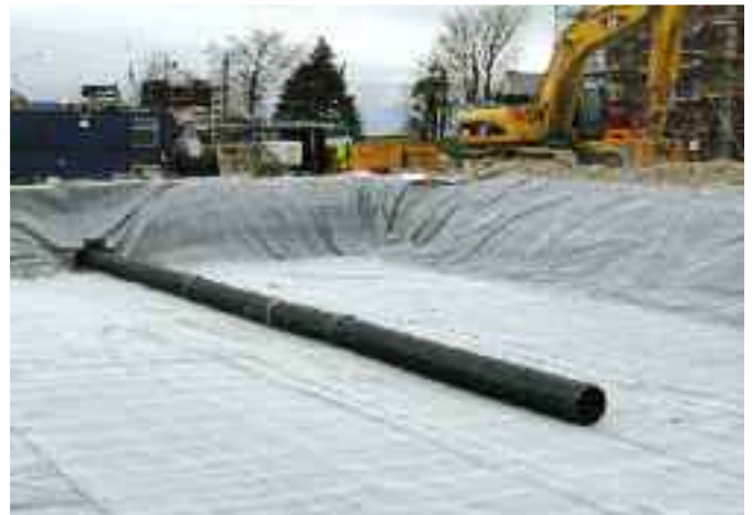
Fig. 4 – Impermeable System Distribution Pipe
