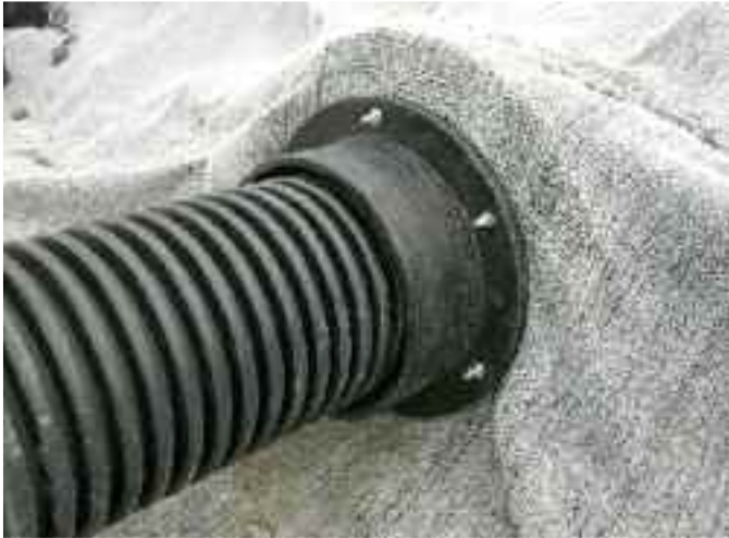
Fig. 5 – HydroSeal Watertight Pipe Joint
