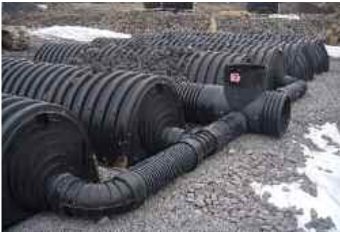
Fig. 14 –Manifold Installation
