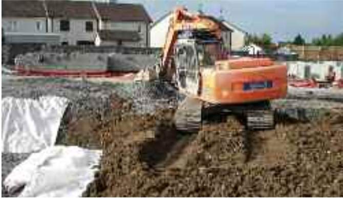
Fig. 19 – Excavator Rutting
