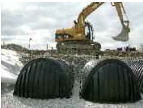
Fig. 17– Track Machine Over Chambers
