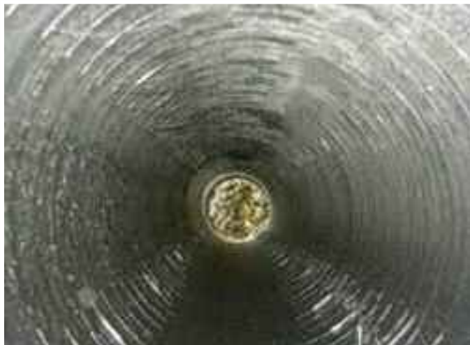
Fig. 24 – Distribution Pipe Inspection
