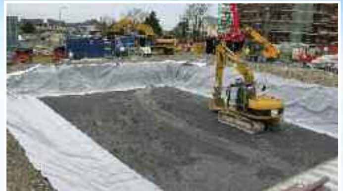
Fig. 2 – Installing GCL Liner
