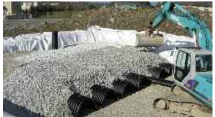
Fig. 18 – Track Machine Working in Base
