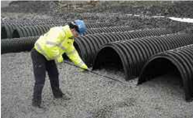
Fig. 10 – Levelling the base
