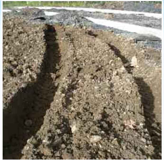
Fig. 20 – Dumper Rutting
