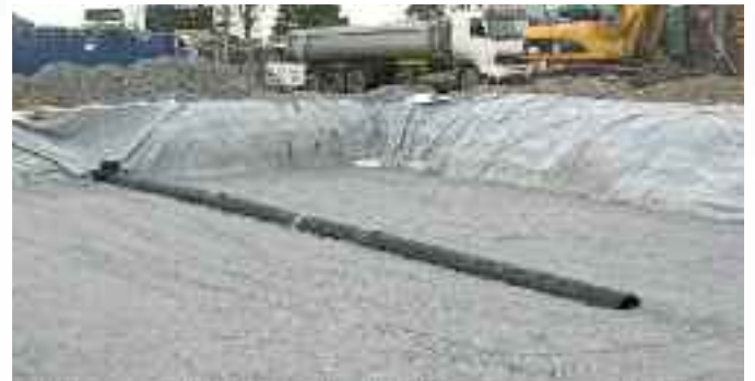
Fig. 6 – Foundation Stone Installed
