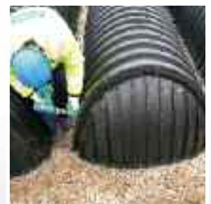
Fig. 10 – Screwing End Cap in Place
