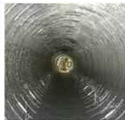
Fig. 14.1 – Distribution Pipe Inspection
