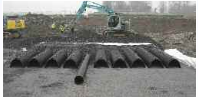
Fig.9.2 – Infiltration /Permeable System
